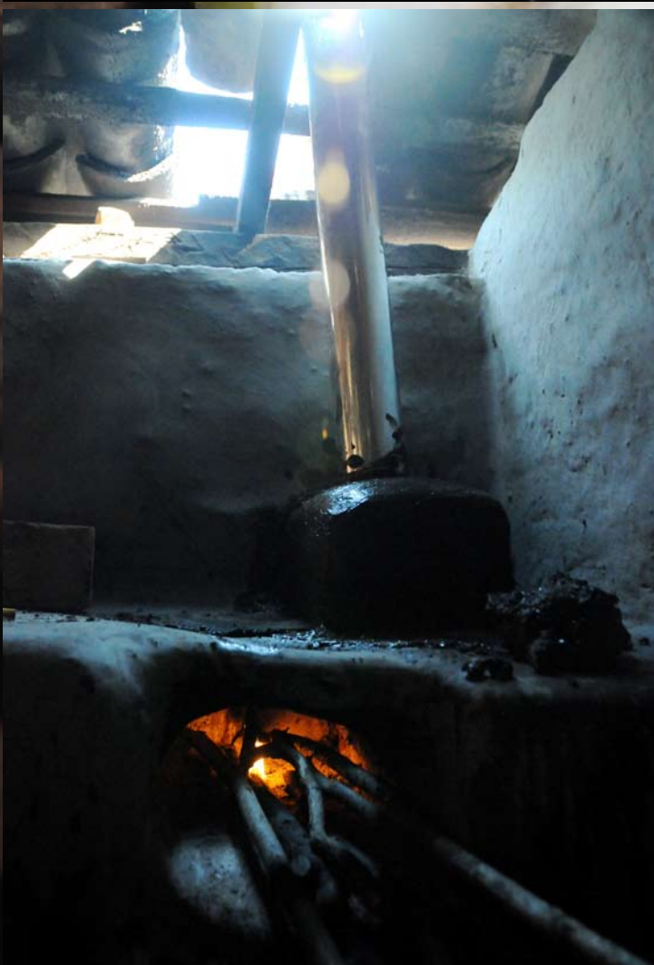
Photos (Top to Bottom): A member of the church helps to install a chimney through the slats of a roof; A wood-burning stove is lit to test a new chimney and help the cement to dry.
